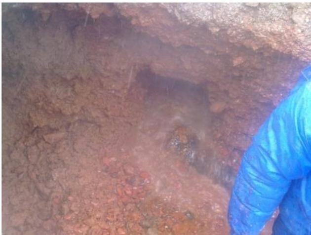
After first circle of measurements and water balance calculation, sound leak detection was conducted. During the detection process, 10 underground leaks and 19 illegal connections were detected.
